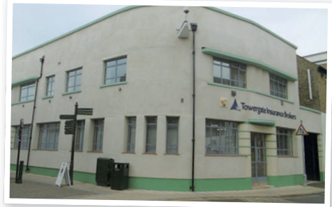
The restored Art Deco façade added to the building that was formerly the Rummer.
